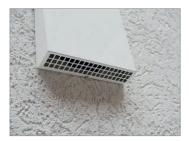
On selecting the installation location, observe the exterior view of the building. In order to harmoniously integrate the devices into the building facade, the devices should be installed at the same height / with the same distance to the windows, for example.
